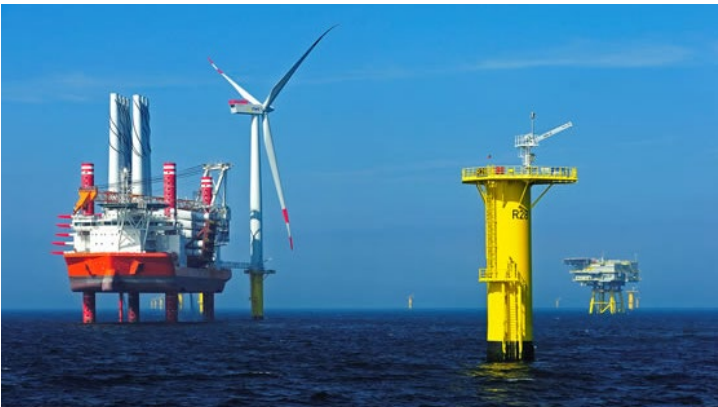
DNV GL studied how integrated design can reduce the cost of off-shore wind generation.
